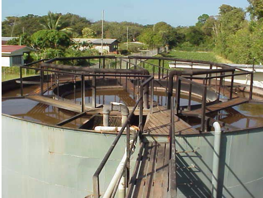
Figure 2A: Photo of Circular Tank
